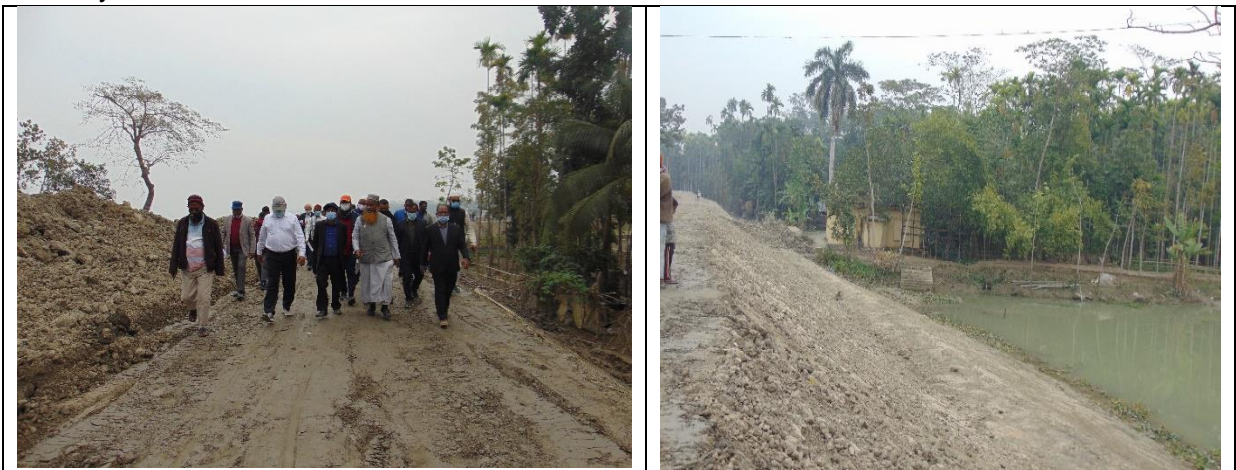
Images 33-34: Embankment construction work
