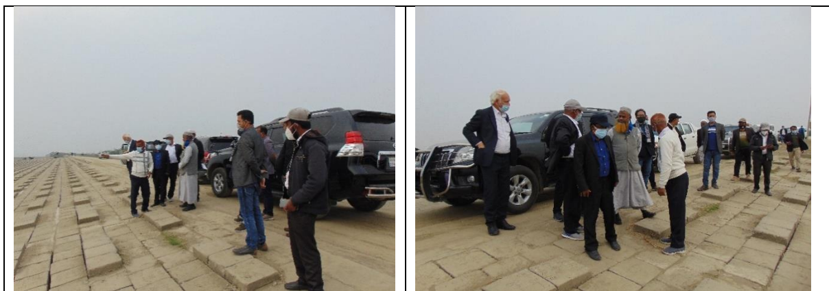
Images 21-22: Slope Protection Works at Km 34+300 to Km 34+878
