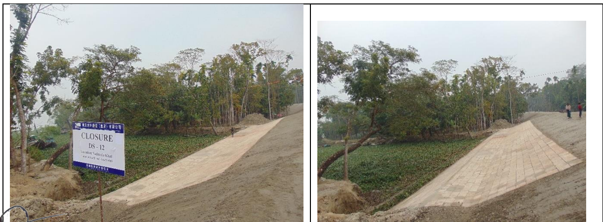
Images 29-30: Closure Construction works
