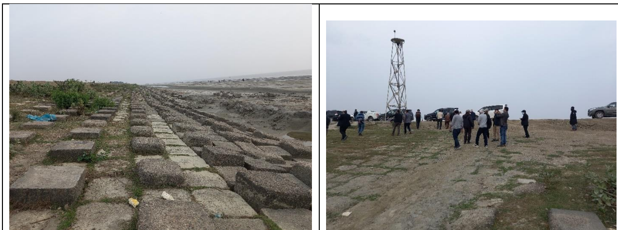
Images 19-20: Slope protection repair works
