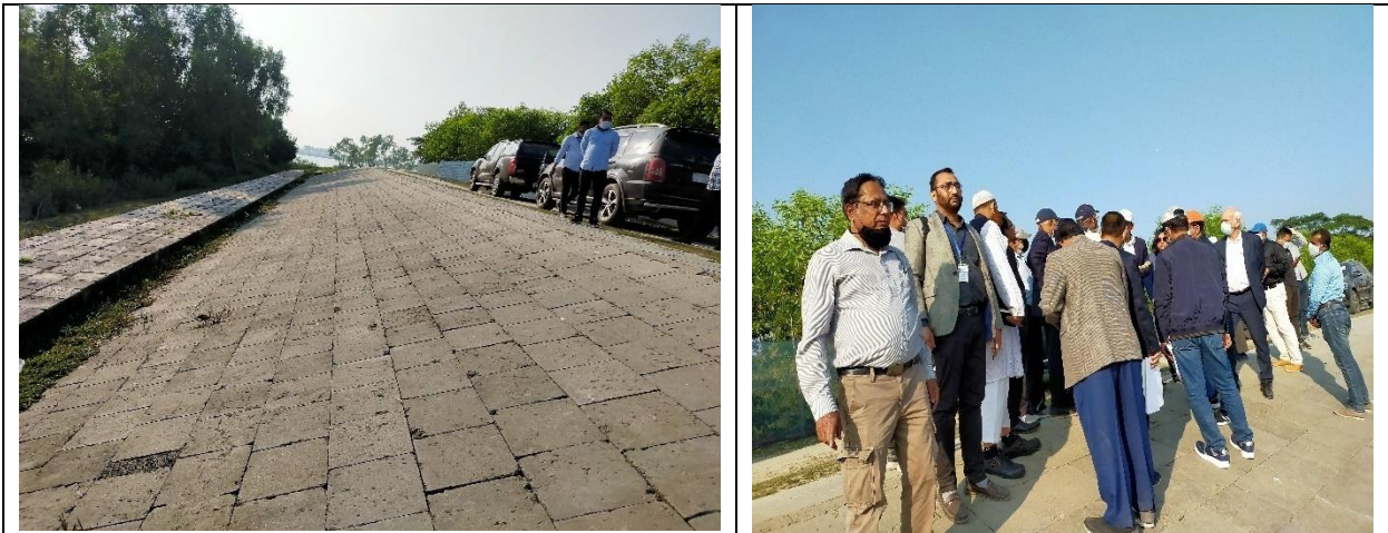
Images 9-10: Slope protection works
