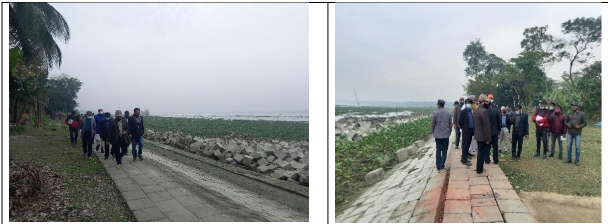
Images 27-28: River Bank Protection Work
