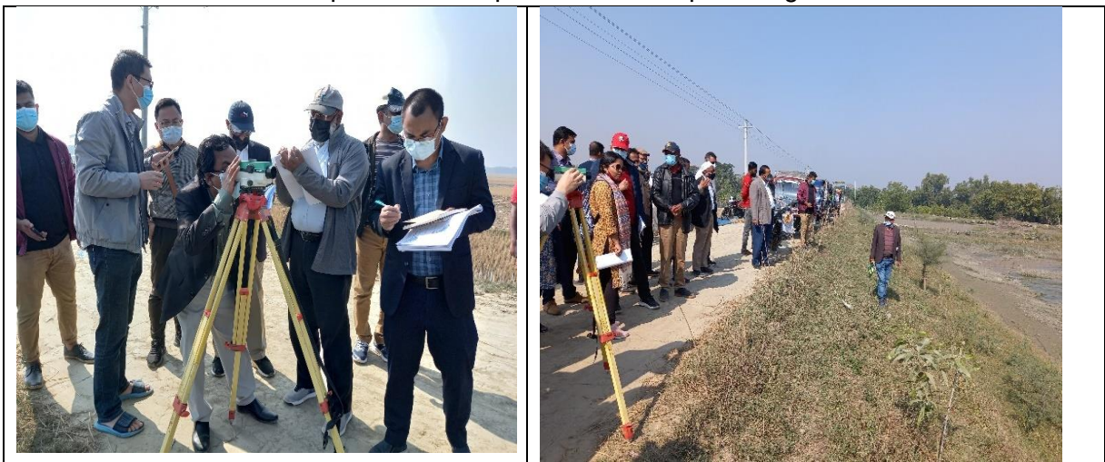
Images 11-12: Measurement of embankment works
